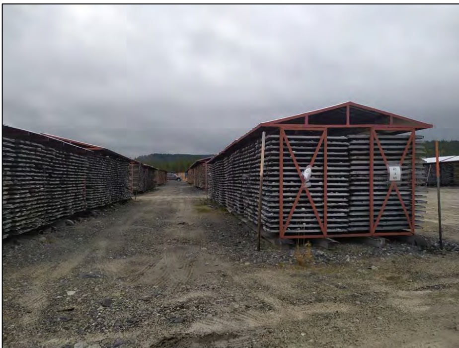
Figure 12-4: Core Storage Area; Core Racks
