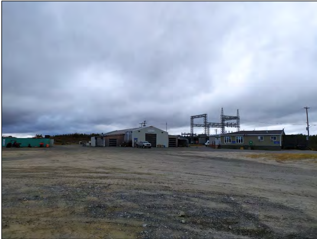
Figure 12-3: Core Logging Facility (centre) and Centre Administrative (right)
